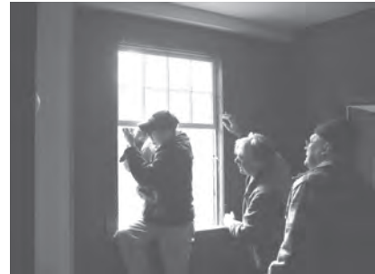
Nick Brennan and John Anderson of Anderson Glassworks install a newly restored window sash on the second floor rear of Seven Hearths.
