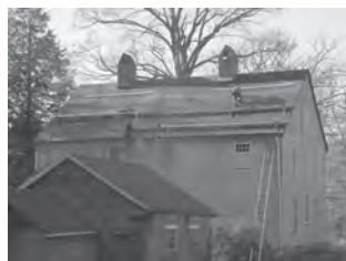
Installation of the Enviroshake roof
