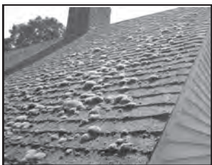
The old roof in 2009
