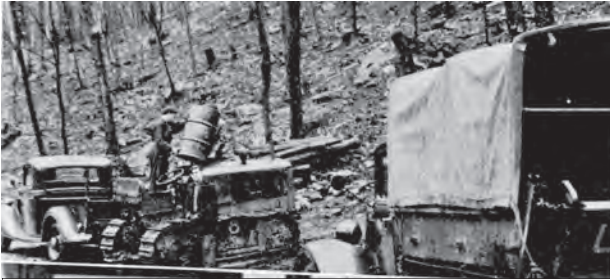
Building the road in Macedonia Photo courtesy of Marty Podskoch
